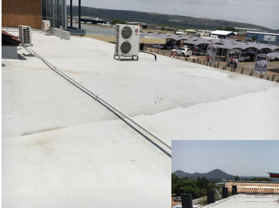
Figure 7: Overview of the lower west-section showing the coating system
