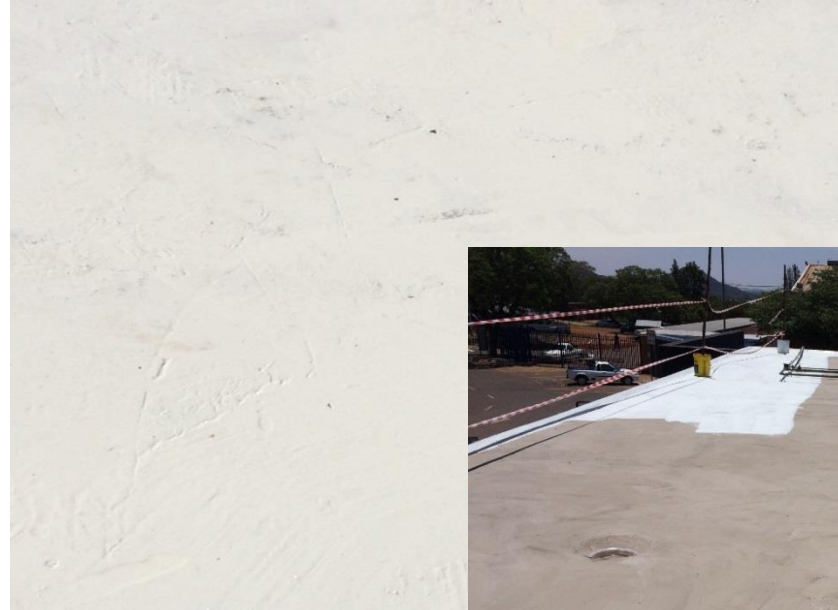
Figure 1: Wonderboom Airport roof after application of the primer
