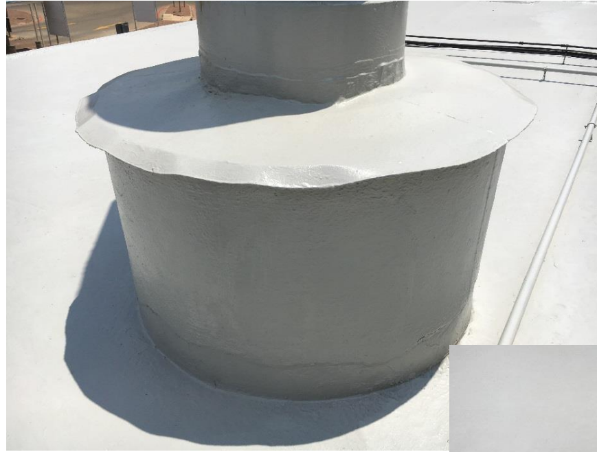
Figure 5: Topcoat showing good finish
