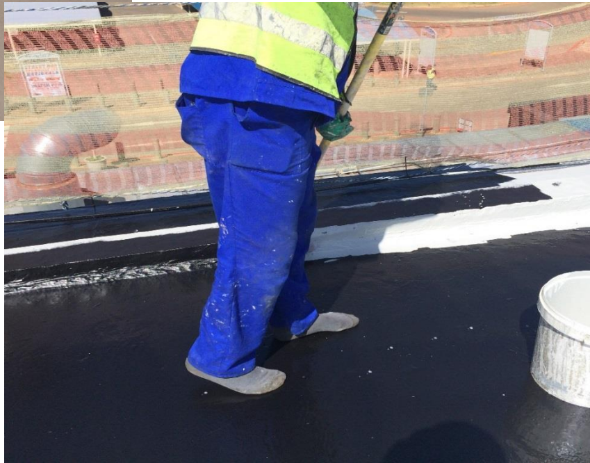
Figure 3: Wonderboom Airport roof during application of the primer
