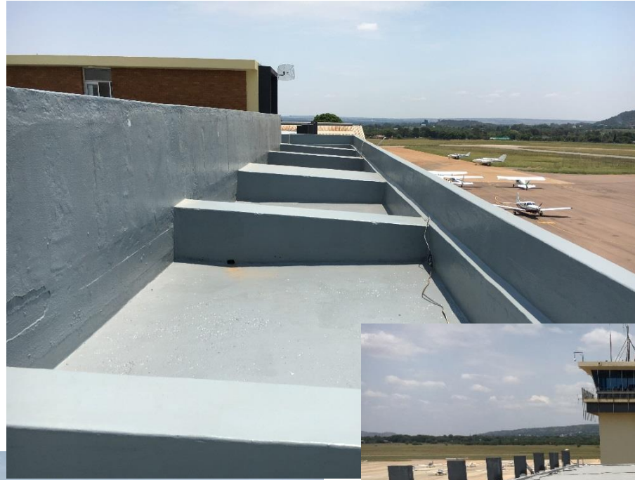
Figure 10: Overview of the upper east-section showing the coating system
