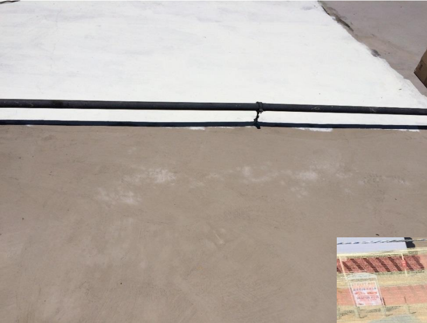
Figure 3: Wonderboom Airport roof during application of the primer
