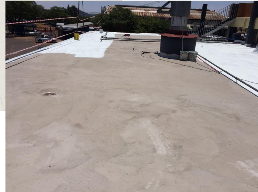
Figure 2: Wonderboom Airport roof during application of the primer
