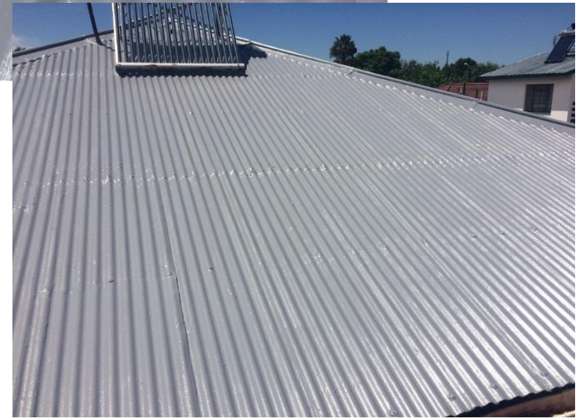
Figure 3: Roof sheet after application of the coating system
