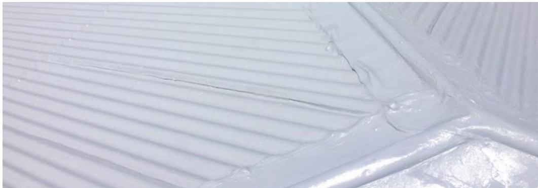
Figure 1: Roof sheet after application of the coating system
