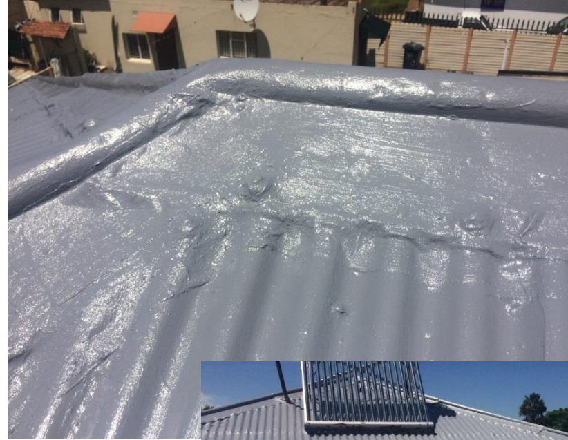
Figure 2: Roof sheet after application of the coating system
